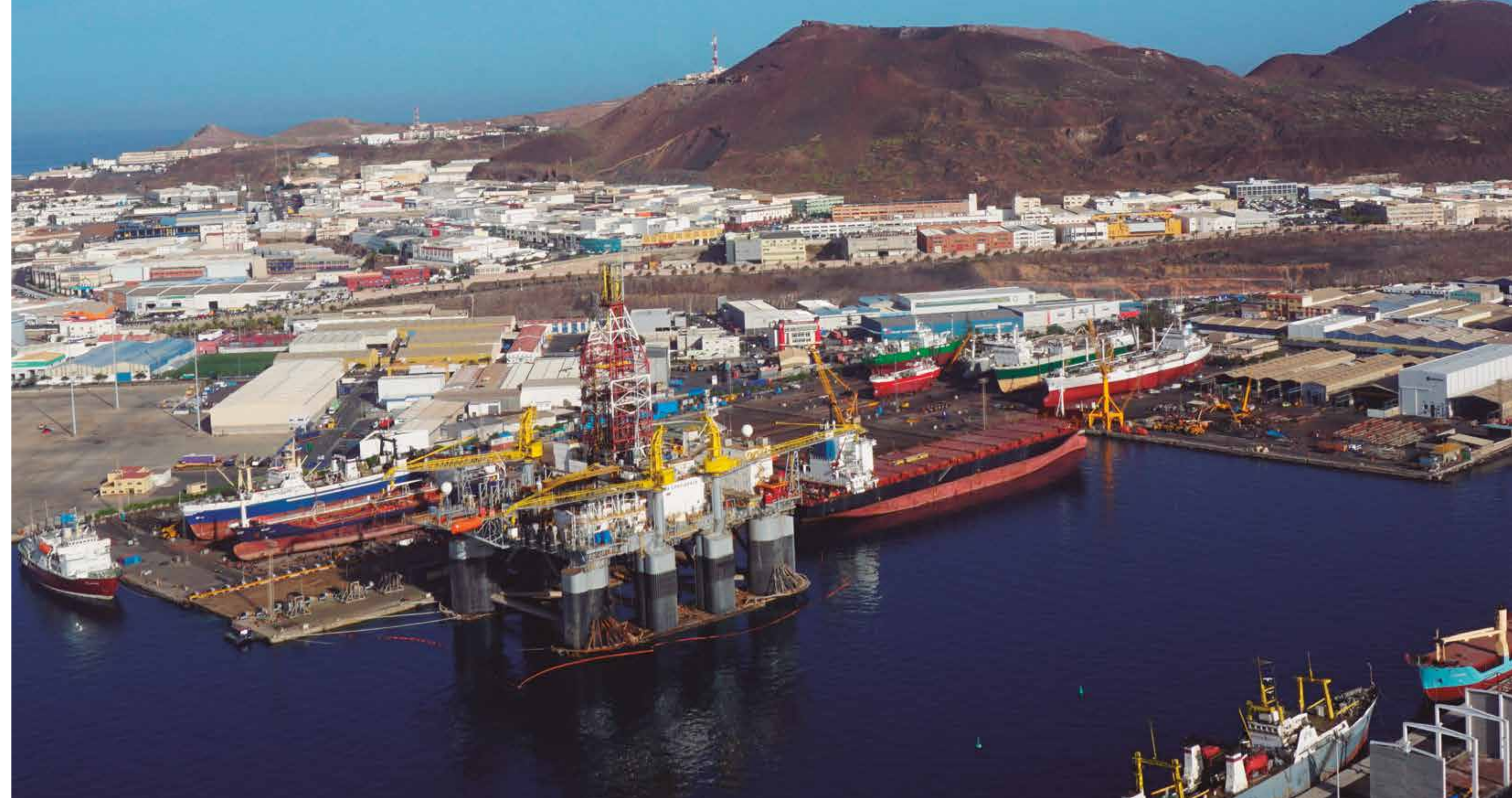
LIFTING PLATFORM OF 175 M LONG AND 30 M WIDE, UP TO 10,000 TONS LIFTING CAPACITY (FOR VESSELS UP TO 36,000 DWT)
